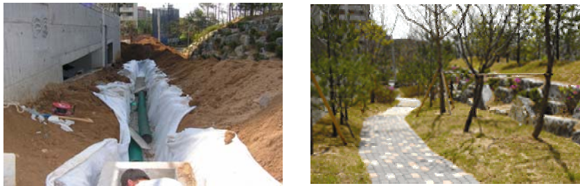
Figure 2. Before and after the application of infiltration barrel and infiltration trench.
